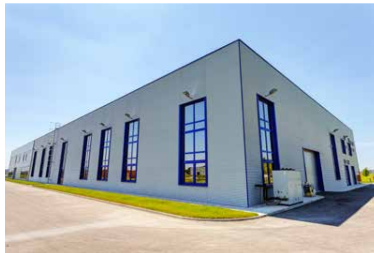
Air handling unit
